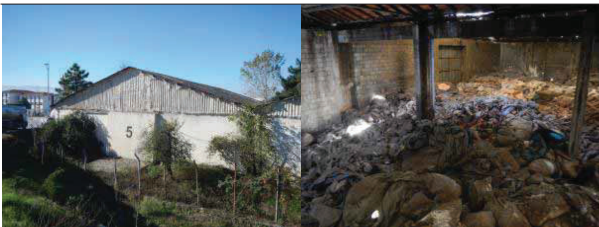
Figure A1.50 Backside warehouse 6 (left) East wall warehouse 6 (right)
