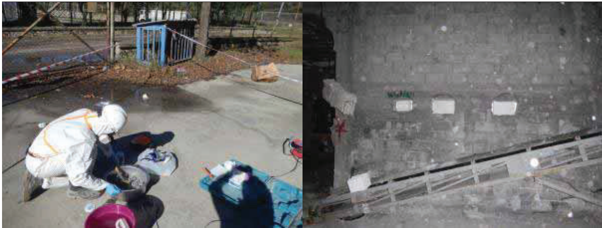
Figure A1.24 Crushing of wall blocks (left) Refilling of holes with new blocks (right)
