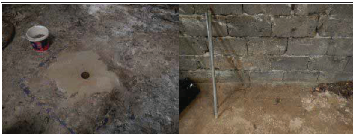
Figure A1.35 Floors (left) First layer concrete blocks (right)
