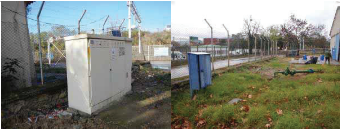
Figure A1.53 Distribution unit outside warehouse 1b (left) Electricity units outside warehouse 4 (right)
