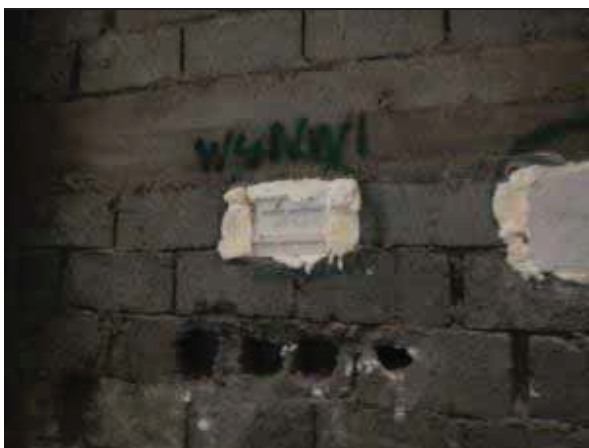
Figure A1.25 Styro foam to close gaps in walls (left)
