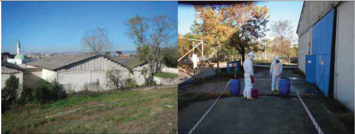
Figure A1.45 Warehouse 3 backside (left) Warehouse 3 front (right)
