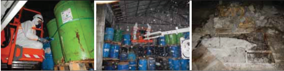
Figure 6 Left and middle binding drums on pallets on top row before moving them for the inventory and right pit filled with POP pesticides and rubble in Warehouse 1
