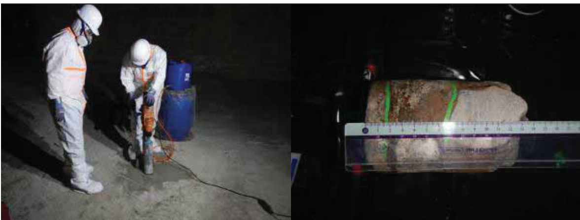
Figure A1.19 Concrete core at W3-F6 (left) Concrete core from W3-F6 (right)
