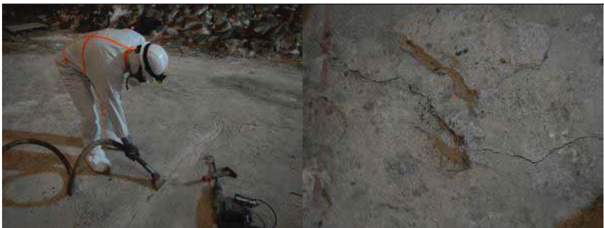
Figure A1.22 Checking cracks in floor (left) Checking the depth of cracks (right)
