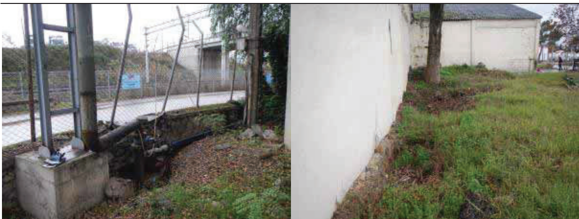
Figure A1.54 Water distribution outside warehouse 2 (left) water collection areas outside warehouse 2 (right)
