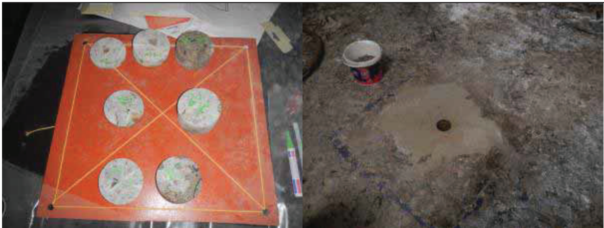
Figure A1.21 Cut concrete cores (left) Refilling with cement (right)
