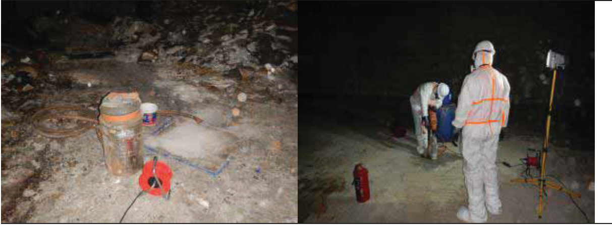
Figure A1.7 Industrial vacuum cleaner (left) Industrial light and fire extinguisher (right)
