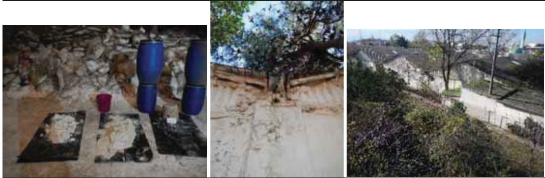
Figure 10 The specific weight measurements of the different kind of POP-pesticides (left dry HCH isomers, dry powder possible DDT and right wet, paste, POP pesticides), middle the blocked and damaged gutter to drain rainwater and right the North-East part of the Warehouse
