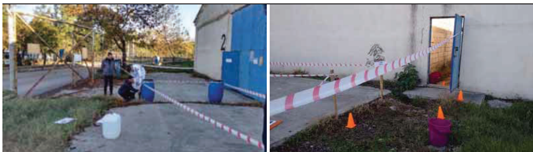
Figure 1 Left the installation of zoning and right the entrance to the de-contamination zone
