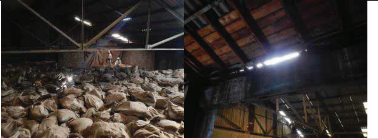
Figure A1.51 Warehouse 6 towards East and South walls (left) Roof of warehouse 6 (right)
