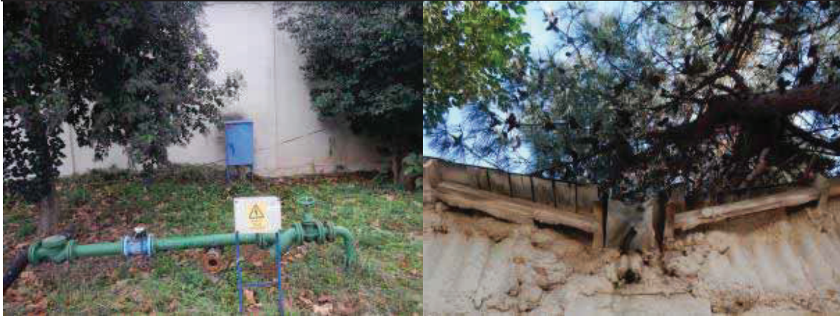
Figure A1.55 Groundwater extraction well at warehouse 6 (left) Blocked gutter between warehouse 4 and 5 (right)
