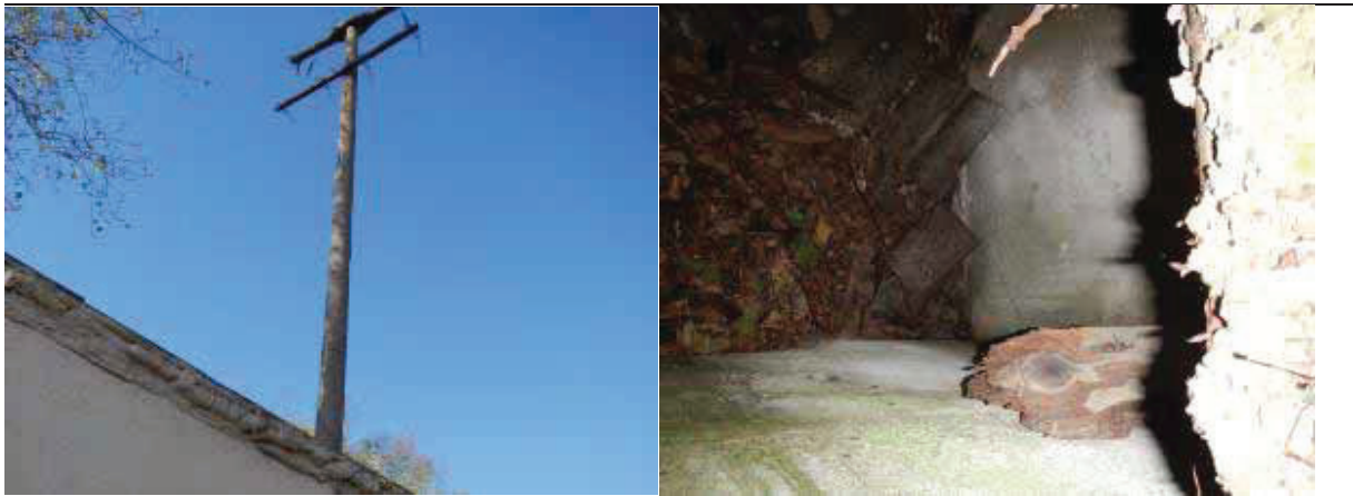
Figure A1.40 Electric pole through roof in warehouse 1b(left) Septic tank outside warehouse 1c (right)
