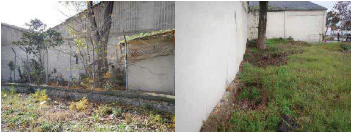
Figure A1.43 Backside warehouse 2 (left) Front of warehouse 2 (right)
