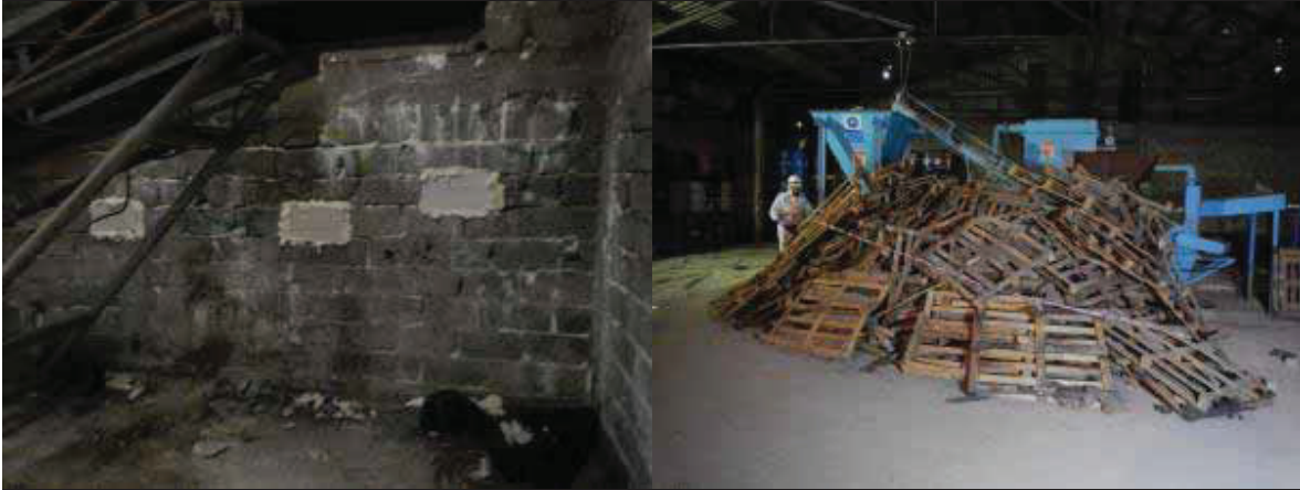
Figure A1.36 Contaminated lower walls(left) Pallet waste (right)
