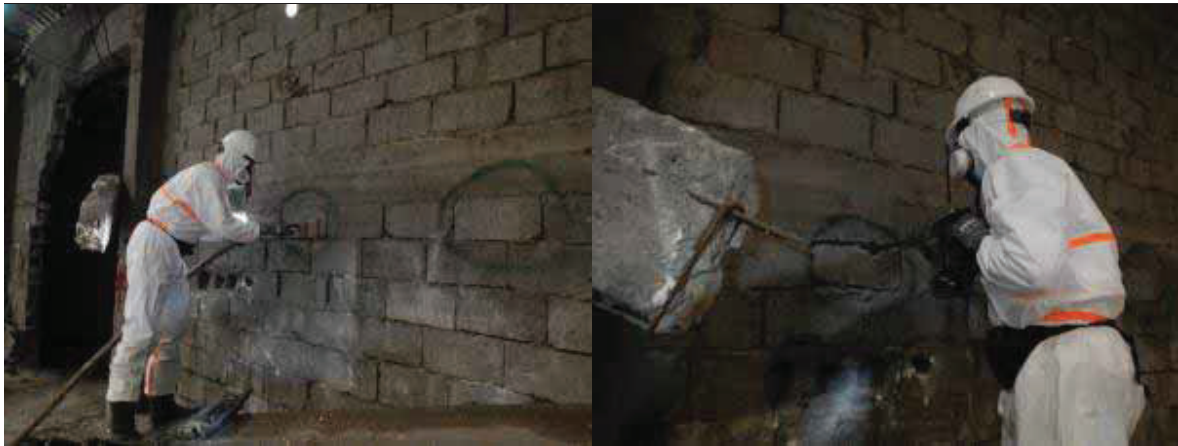
Figure A1.23 Cleaning of blocks with vacuum cleaner (left) Removal of blocks from the wall (right)
