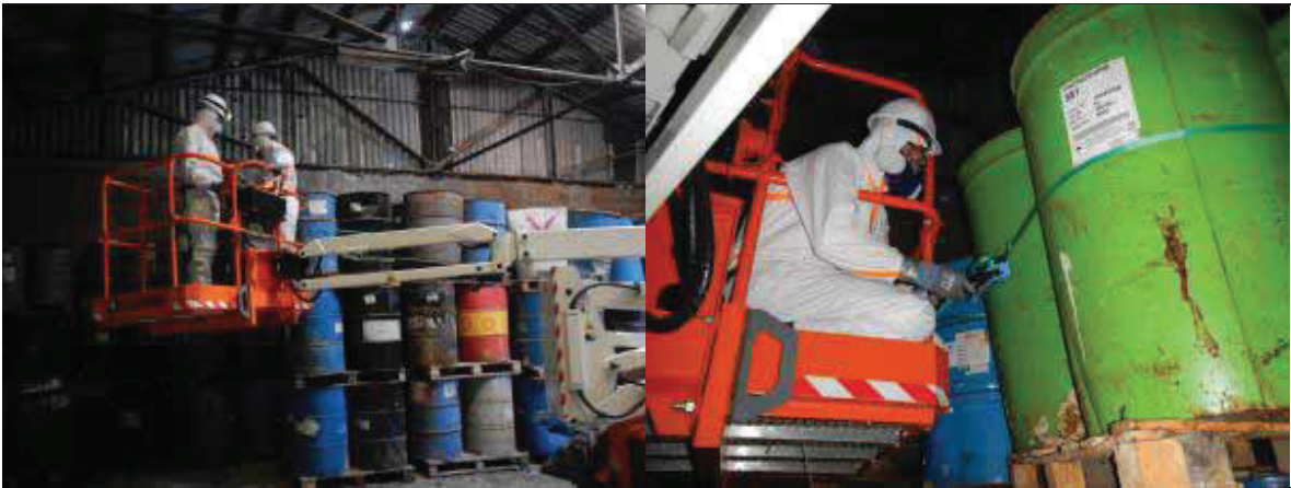
Figure A1.11 Binding of dangerous drums (left and right)
