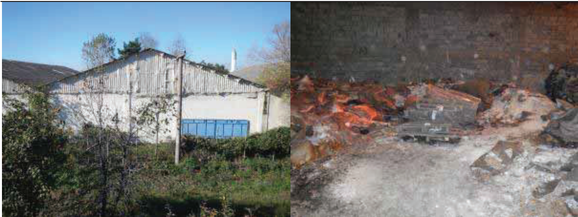
Figure A1.49 Backside warehouse 5 (left) Back wall warehouse 5 (right)
