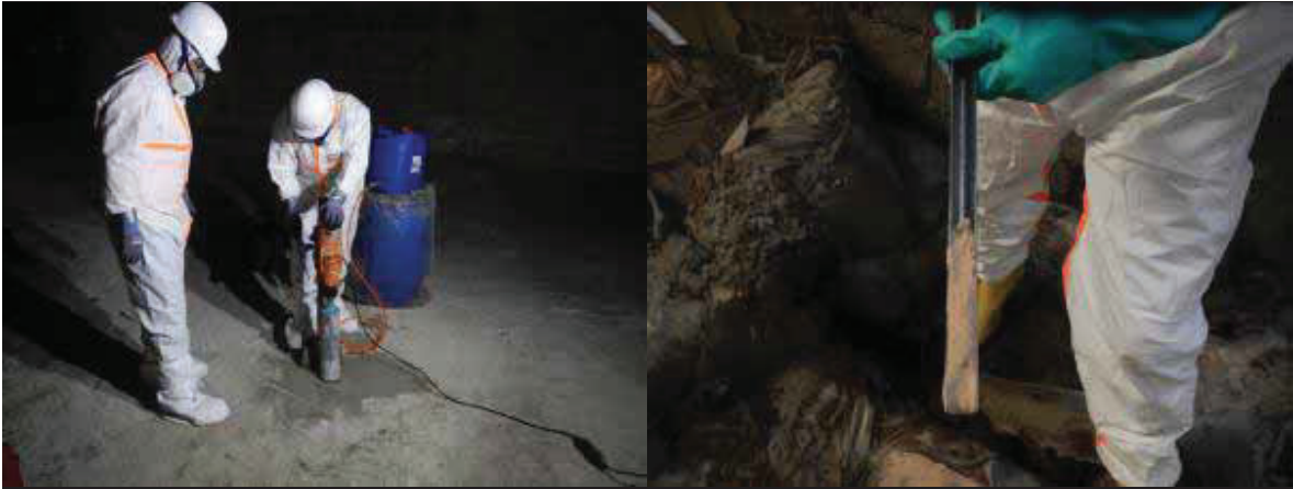
Figure A1.5 Concrete coring (left) waste sampling equipment (right)
