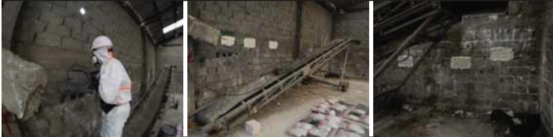
Figure 9 right removing building block from wall for sampling, middle the repaired clean sample locations and right the repaired contaminated sample locations
