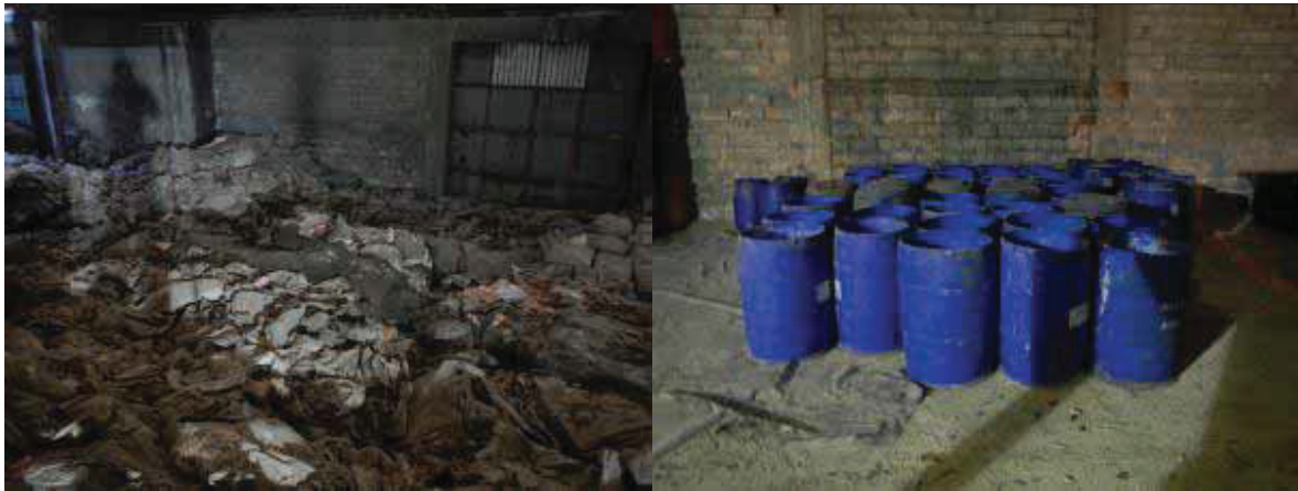
Figure A1.33 Empty packaging in warehouse 4 (left) PE drums (right)
