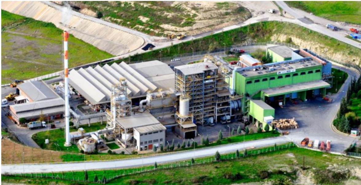
Figure 1: Overview of the IZAYDAS Incineration Facility
