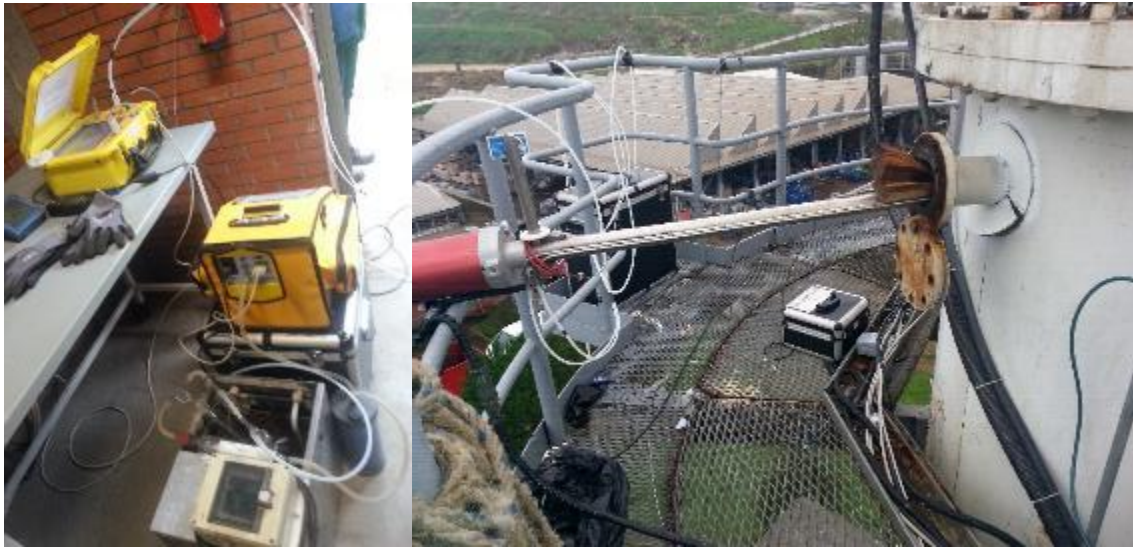
Stack gas emission sampling
