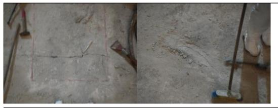
Figure 8.1 Large cracks in site floors (warehouse 4)
