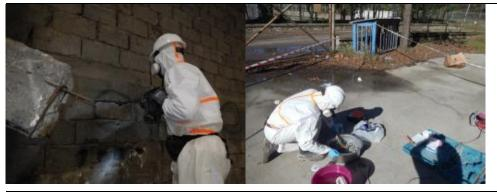
Figure 5.6 Collection of building blocks (left) Outside processing of blocks prior to transfer to laboratory (rigth)
