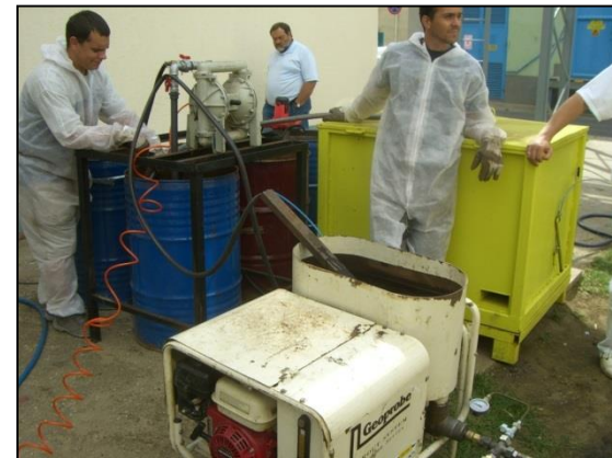
Figure 23: preparation of ARDEC mixture on site
