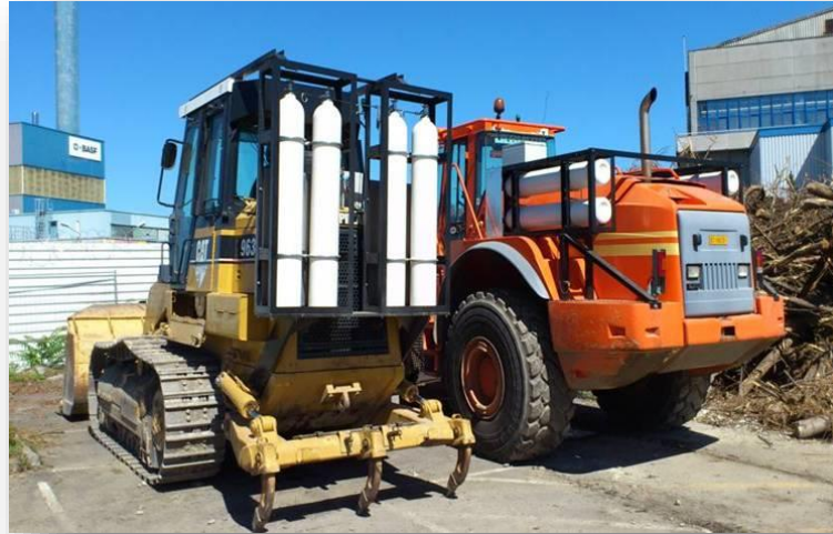
Drivers' cab pressurization with breathable air injection : 15 machines are equipped Special pressurized trucks on site
