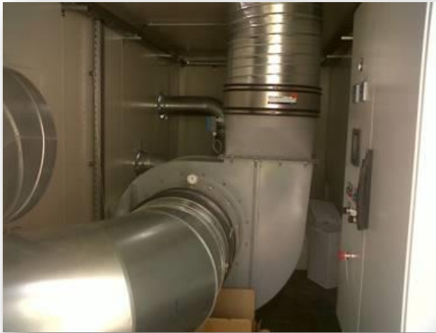
Air extractors : 40 000 m 3 /h Associated air treatment
