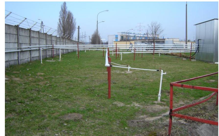
Barrier air-sparging and bio-slurping southern boundary
