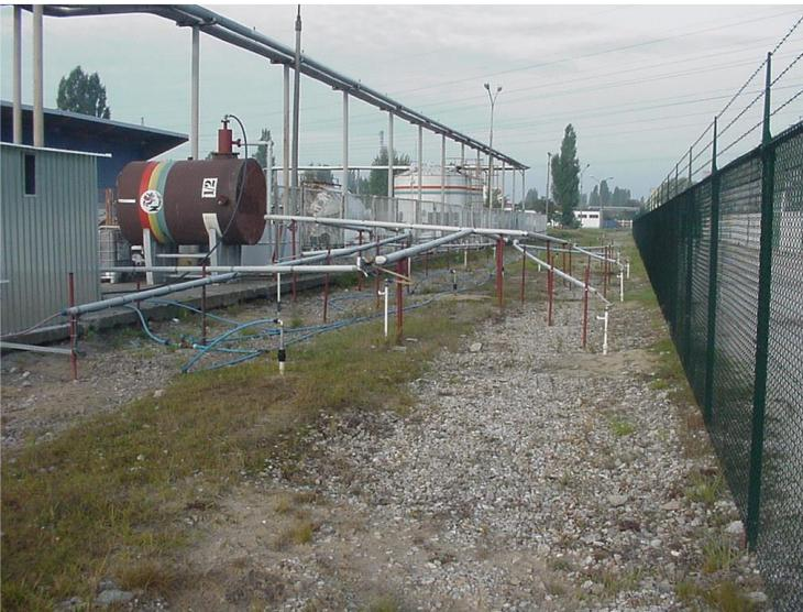
Barrier air-sparging and bio-slurping northern boundary
