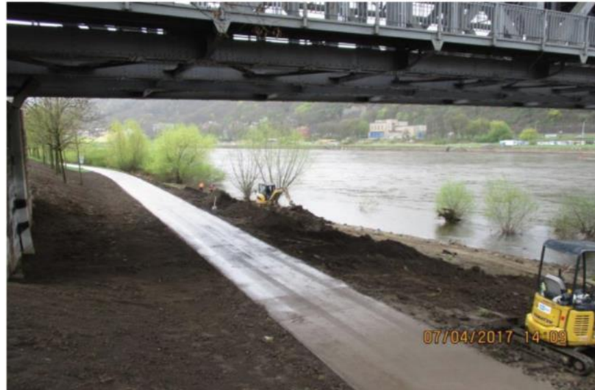
Photo: Site works
