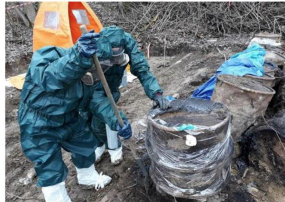
Photo: Removal of hazardous waste from an underground storage
