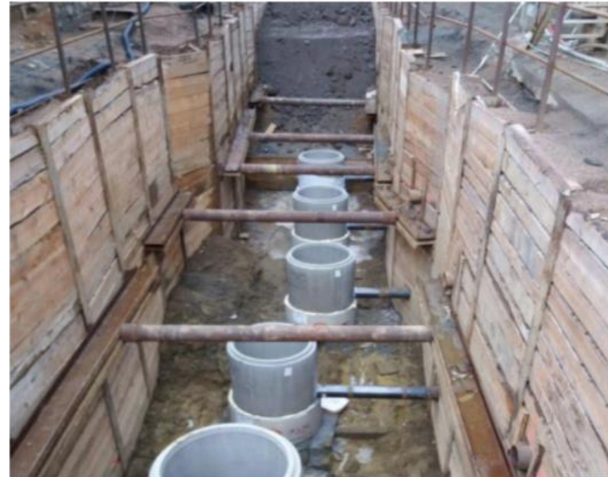
Photo: Site works
